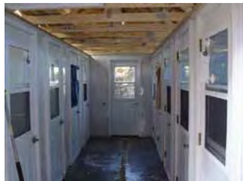
The sloped floors and central drain help keep the animals clean and comfortable.
